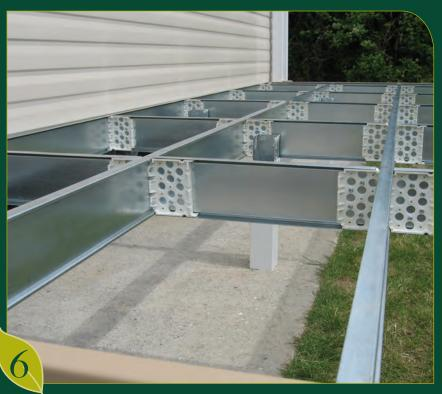
The steel sub-frame is simplicity itself. It consists of just two components - a steel 'I' beam and its connector. The sub-frame is easily connected into a grid pattern and the deck boards are fixed directly to the steel joists.
